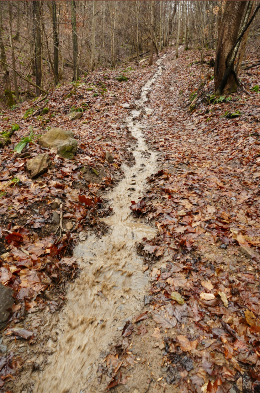
Unsustainable trail construction practices can lead to costly damage from erosion and runoff, as is seen here on a motorized trail above Coeburn, Virginia.
